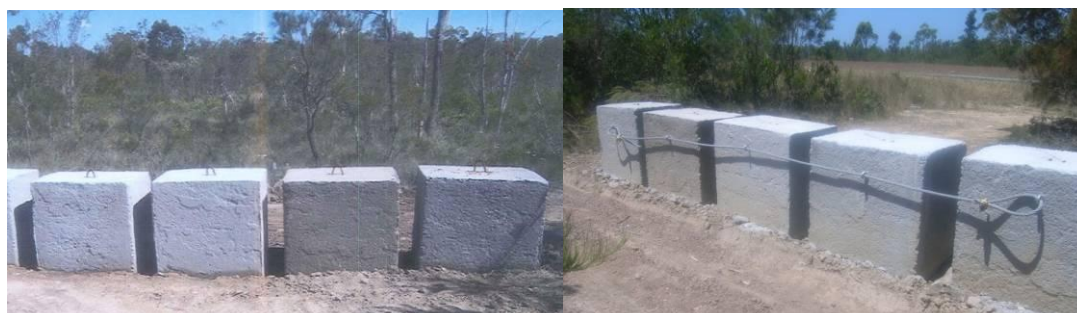
Figure 4: Blocks in place (left) and blocks with cable joins (right).
