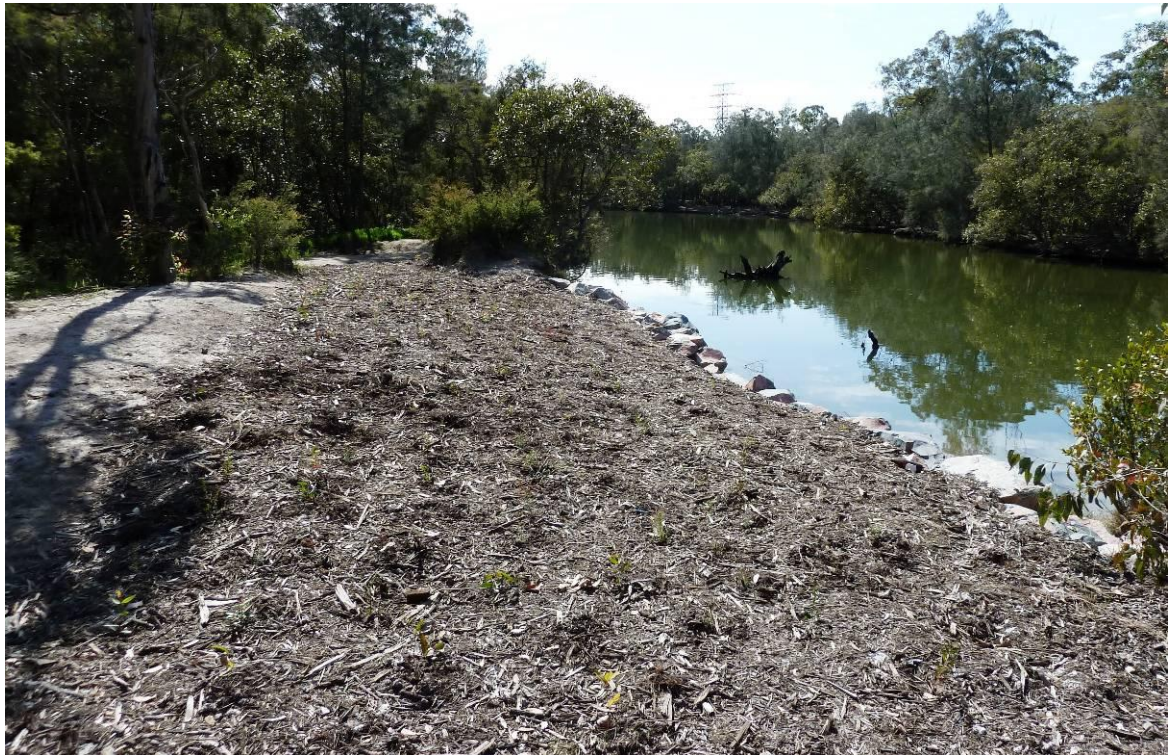
Figure 7: Revegetation and mulching along rock stabilised creek bank.
